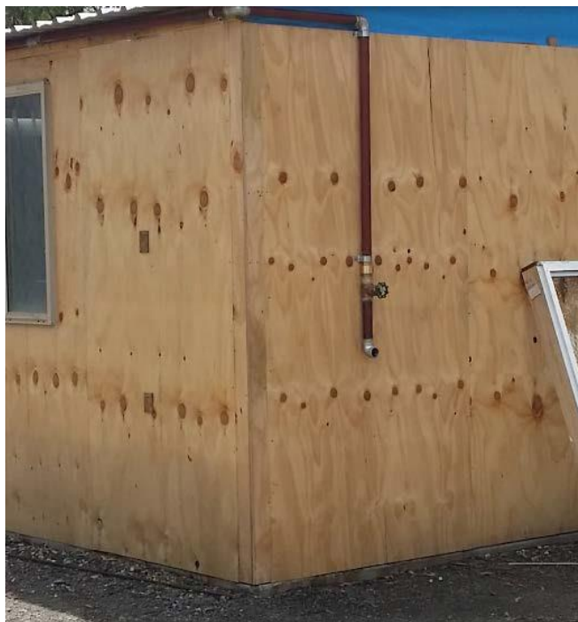
Figure 16: Residential Sprinkler System External Fitting
